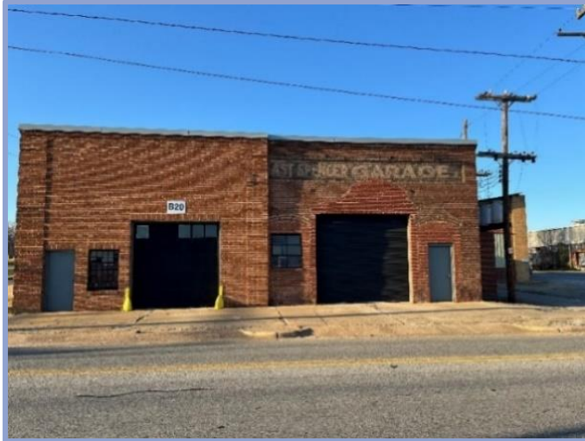
Figure 5: Vacant Auto Service Facility No Longer in Operation
